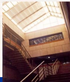
▲ The roof of the solar chimney is of low e-glass. A 25-kW peak solar photovoltaic system has been installed on the roof
