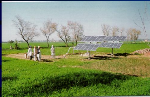
An SPV Water Pumping System installed at Murad Nagar, Ghaziabad, Uttar Pradesh
