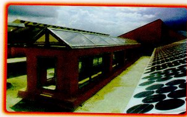
▲ The roof of the solar chimney is of low e-glass. A 25-kW peak solar photovoltaic system has been installed on the roof
