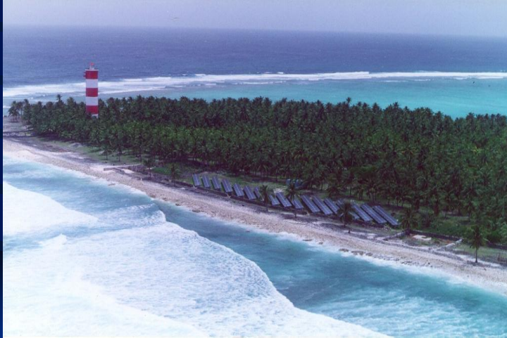
100 kW PV Power Plant at an Island in Lakshadweep
