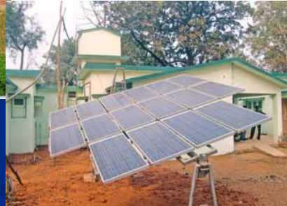
An SPV Water Pumping System installed at Murad Nagar, Ghaziabad, Uttar Pradesh
